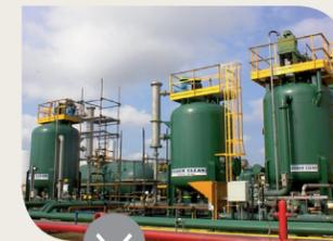
**POWER CLEAN™** nutshell filters are effective for the removal and treatment of hydrocarbons and suspended solids from produced water applications.
