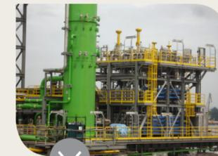
The **SULPHATE REMOVAL PLANT (SRP)** is used to extract sulphates from seawater prior to injection. The SRP uses nano-filtration membranes to remove sulphates while leaving the other salts unaffected, thus maintaining the stability and permeability of the formation clays.
