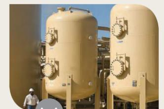
**ID ION EXCHANGE SOFTENING** High specification Strong Acid Cation (SAC), Weak Acid Cation (WAC) or a combination of both in series, or a multi-step process of softening with other water treatment technologies for produced water treatment.
