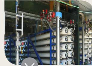
**OPUS® II** technology is the next generation OPUS process that utilizes Ceramic Ultra-Filter membranes as pretreatment prior to ion exchange and reverse osmosis operated at an elevated pH. The effluent is high quality water suitable for industrial reuse or surface discharge.
