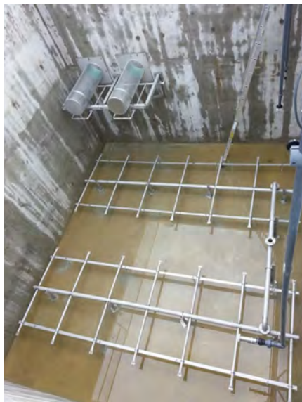
Moving bed biofilm reactor showing aeration grids and retention sieves (left) and steady state operation (right).
