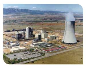
Based on the PRENFLO™ gasification process, the plant uses a mixture of local coal (from ENCASUR) with a high-ash content and petroleum coke produced at a nearby REPSOL refinery as feedstock.
