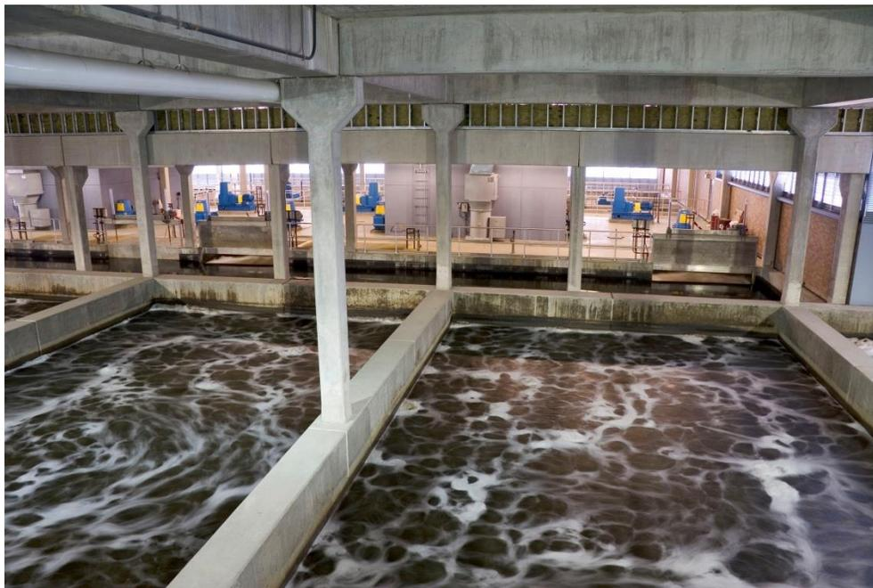
*Figure 1: Top view of BIOSTYR<sup>®</sup> cells at 84 MGD facility*
