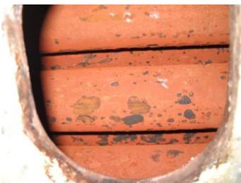
Annual boiler inspection reveals deposit removal on tube surface & presence of Magnetite surfaces
