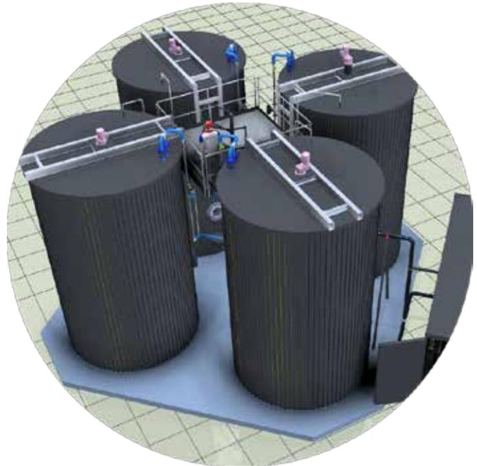
In addition to being the first Biofarm this ANITA™ Mox plant was designed to treat up to 200 kg NH<sub>4</sub>-N/d with 85% total nitrogen removal and 95% ammonia removal.
