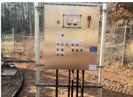
Dedicated control system with Intelligent programmable relay (Zelio) or PLC with HMI. All automatic sequences of operation, manual operation, protections and alarms included. Local control station for tests and maintenance (if applicable). Standard control system and custom system upon client standards are available. Design and engineering by Veolia.
