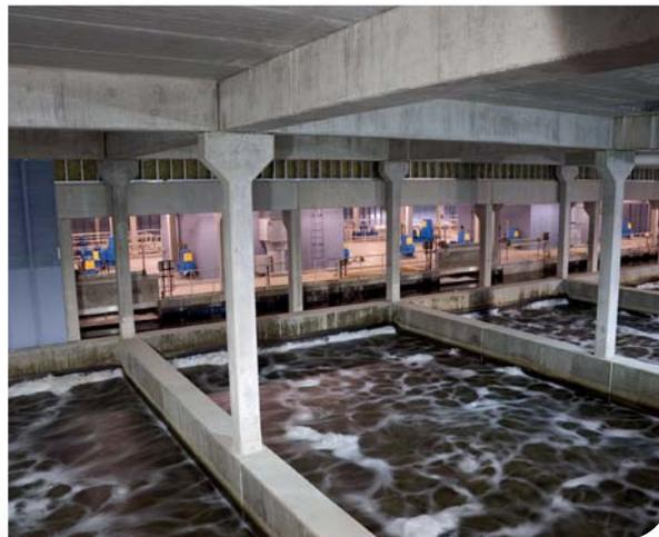
*Treated effluent at top of cells*
