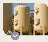
ID ION EXCHANGE **SOFTENING** High specification Strong Acid Cation (SAC), Weak Acid Cation (WAC) or a combination of both in series, or a multi-step process of softening with other water treatment technologies for produced water treatment.
