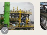
The **ROSS**™ System is a simplified, yet robust solution for the treatment of oilfield produced water. Ceramic Ultra-Filter membrane technology, this system provides removal of oil and silica as well as softening of the water simultaneously in a fully modular system.
