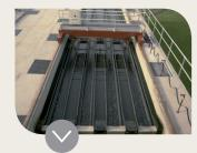
The **MULTIFLO**<sup>™</sup> process can be used in clarification or water softening applications. The proprietary Turbomix reactor promotes formation of heavier solids. The system combines coagulation, flocculation, and lamella settling in a single unit.
