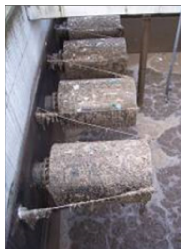
Consequence of poor screening prior to an MBBR process: clogging of outlet sieves.
