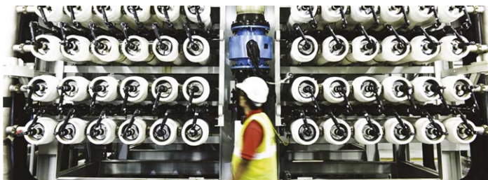
Figure 3. Membrane technologies can offer lower OPEX and energy costs than thermal technologies, but these solutions require pretreatment and chemical cleaning.
