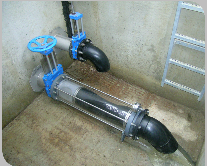
Figure 1: Typical Installation, HYDROVEX® TTT
