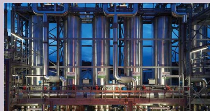
**Exelys™** and **BioThelys™** are both high solids thermal hydrolysis solutions. While Exelys™ is a fully continuous process, BioThelys™ is a continuous batch process. Both processes utilize high temperature (310 to 330 °F) and pressure (85 to 100 PSIG) to sterilize sludge which is retained (SRT) for 20 to 30 minutes at these conditions:
