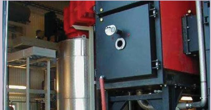
Additionally, the BioCon™ dryer can be fueled by the biosolids end product by incorporating the ERS which can result in an autogenous system by combusting the end product and utilizing the heat of combustion to fuel the dryer.
