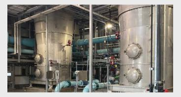
Upon extended exposure to hard water, calcium and magnesium deposits may form on the interior of pipes and other surfaces. This accumulation is most common in areas where water is being heated, and might threaten to block water flow, which could in turn cause reduced efficiency or complete failure. Water softening systems reduce water hardness to prevent scale build up and improve drinking water taste and aesthetics.
