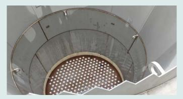
Actina™ reduces calcium hardness, metals and other contaminants with a simple, fluidized bed reactor that uses a catalyst (sand, pellets) to promote calcium carbonate precipitation. A strainer plate is located at the bottom of the reactor and is specifically designed for pellet softening that allows for material in raw water to pass. Caustic/lime plus softened carrier water is pumped to a removable chemical dispersion unit for pH adjustment.
